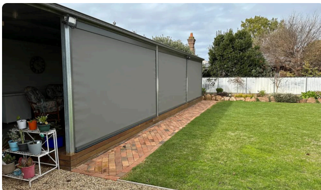
Outdoor screens, Riverina. Client's own job photo.
